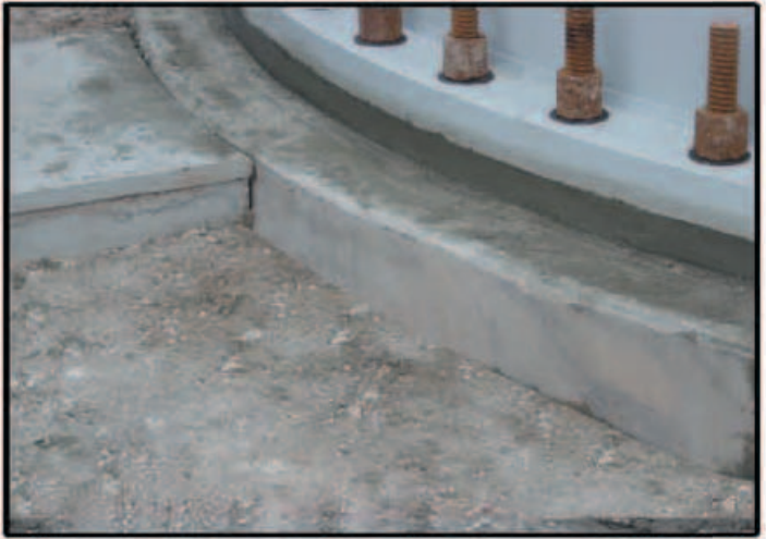
Finished V-1 Grout installation on large equipment ring.
