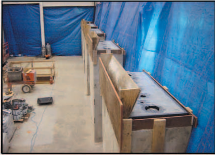
Multiple sole plate forms for V-100 Epoxy Grout pour.
