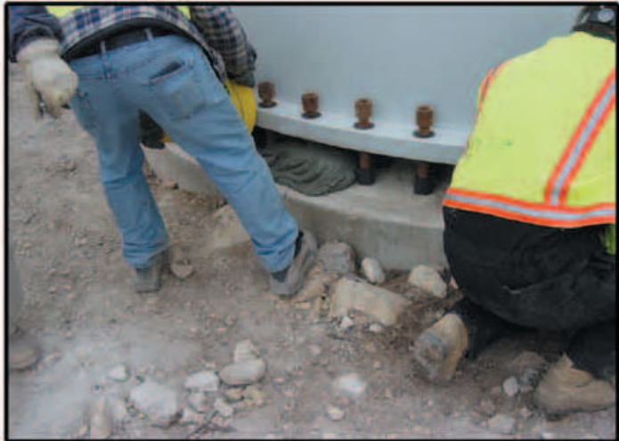
Placing V-1 Grout for large equipment ring.
