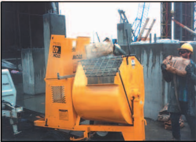
V-1 Grout mixed in a power grout mixer.
