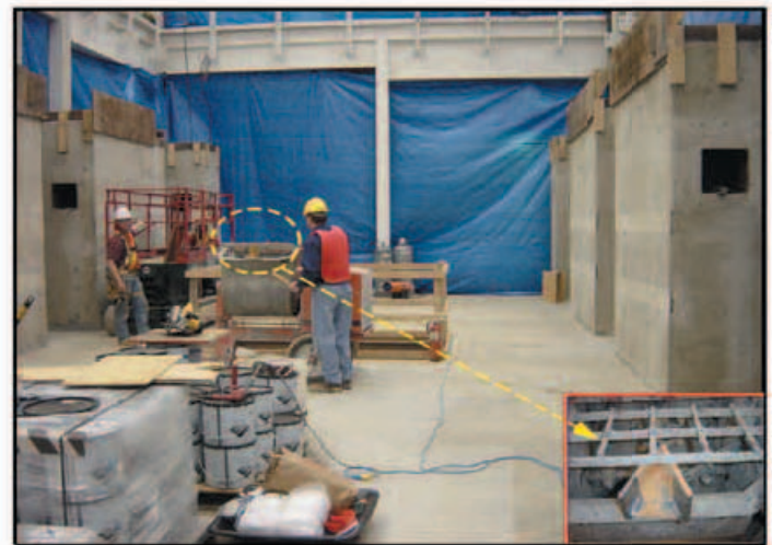
V-100 Epoxy Grout mixed in a paddle type power mixer with a two-bucket divider.
