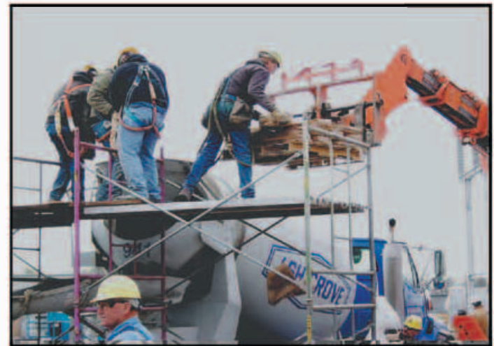
V-1 Grout mixed in a cement truck.
