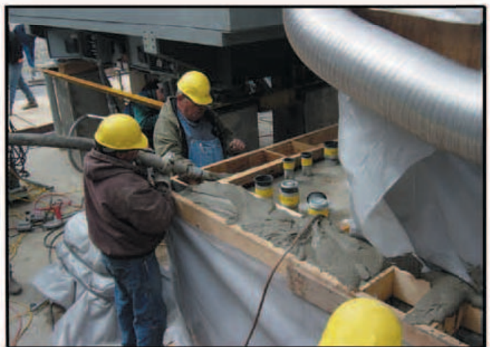
Pumping V-1 Grout on a large turbine generator project.
