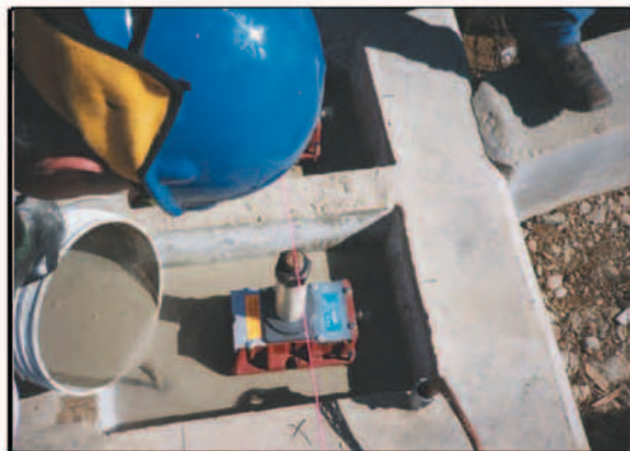
Pouring V-1 Grout for a power generation Fixator application.
