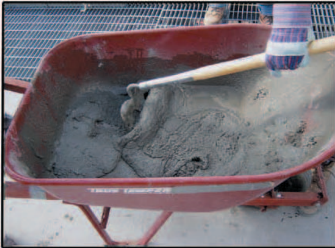
V-1 Grout mixed in a wheelborrow with a hoe.
